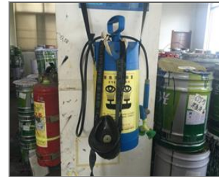
Photo of the sanitary facilities eye washing machine.JPG
